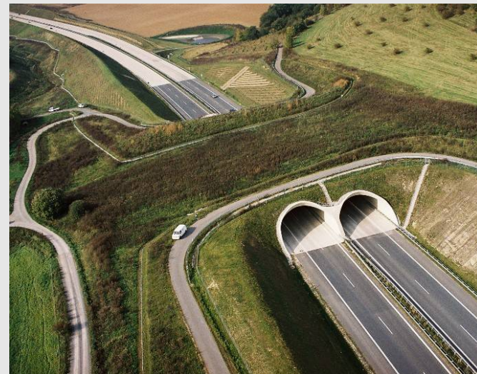
Picture No. 13: Ecological bridge “Landschaftsbrücke Meuschaer Höhe” crossing required to protect environmental use of landscape by wildlife Steel-concrete bridge, practically a tunnel, section 90 m
